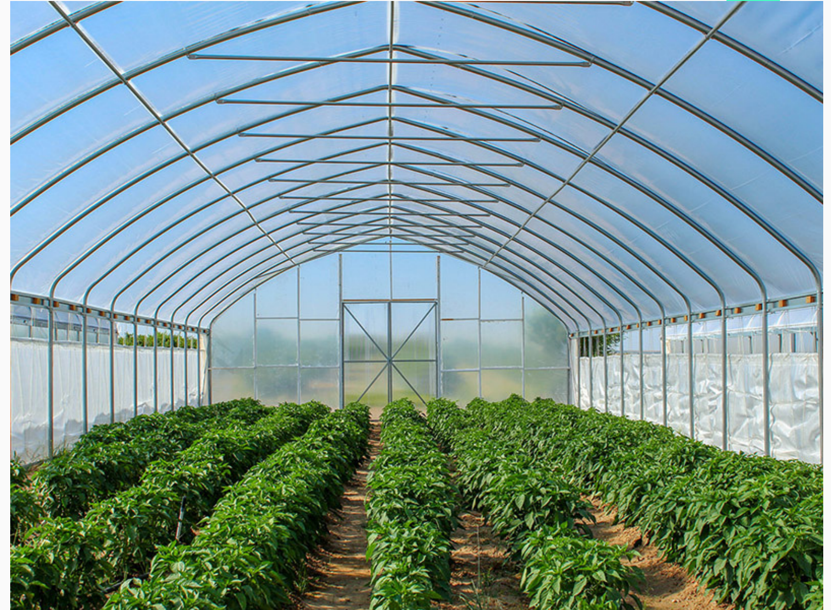
NAPI CHILI PRODUCTION GREENHOUSE
