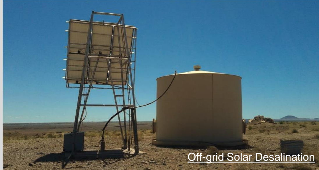
Cutter Lateral Water Treatment Plant
