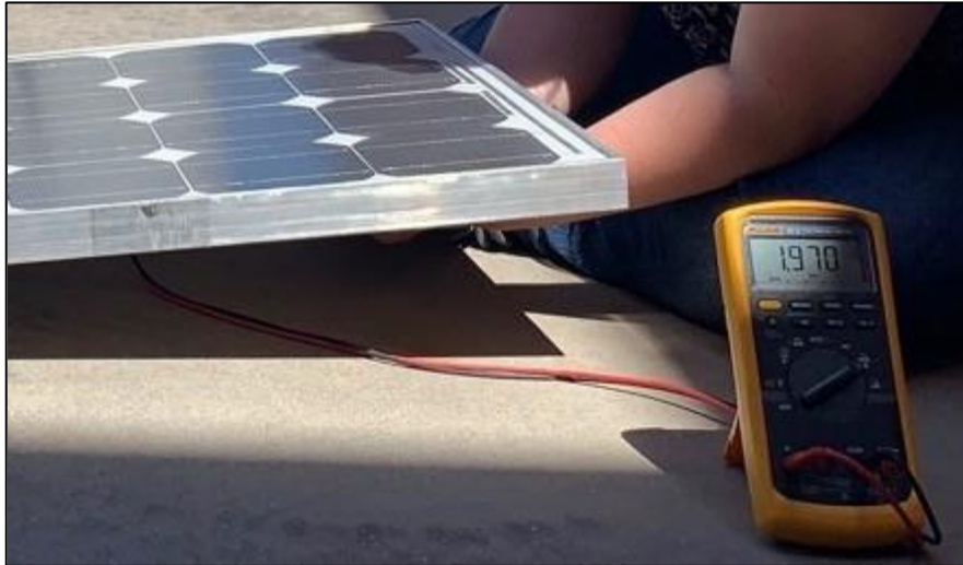
Current measurement of a completely illuminated PV panel reading 1.97 A
