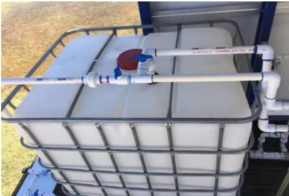
Figure 5. Lines returning flow from either the NF canisters (P5a upper pipe carrying concentrated reject flow) or prefiltration units (P5b lower pipe) as they reenter the raw water (feed) tank from the top. Valves are positioned for the three normal modes of operation in which brine is recycled to the feed tank (both V5a (top, right) and V5b (lower left) are closed). ii.
